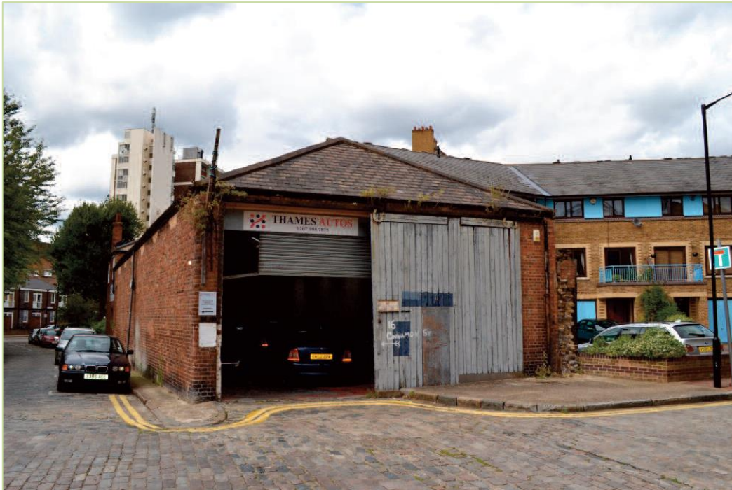
Figure 10: Site C – building used as a garage
